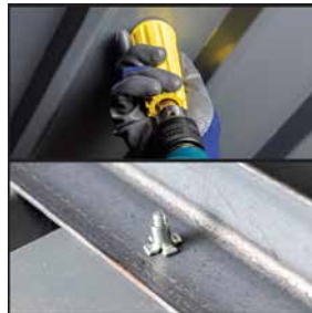
4. Install by Expanding Anchor
