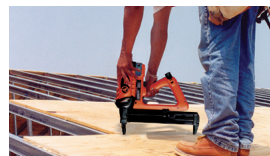
Plywood attachment —using TrakFast plywood to steel pin
