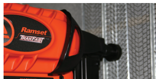
Lath attachment - using one-inch TrakFast discs and magnetic probe adapter
